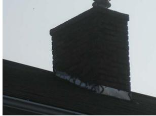
• Improve: A rain cap and vermin screen should be installed on the masonry chimney.
