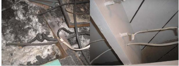
• Improve: Any knob-and-tube wiring that is exposed during renovations should be replaced.
