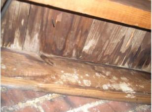
• **Monitor:** Prior repairs to the roof structure (plywood sheathing) are evident in the attic. It may be wise to consult the current owner regarding their knowledge of the roof structure and/or any repairs that became necessary.
