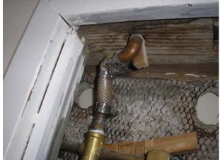
• Monitor: The supply piping shows evidence of prior leakage in the kitchen.
